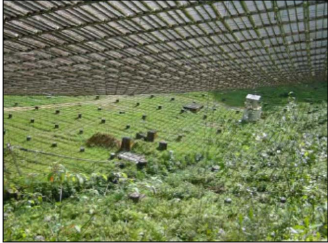
View underneath the primary reflector showing the tieback cables and concrete blocks
