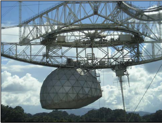
Suspended platform with azimuth arm supporting the radome (left) and line feed receiver on the right. The secondary and tertiary reflectors and horn feeds are housed within the radome
